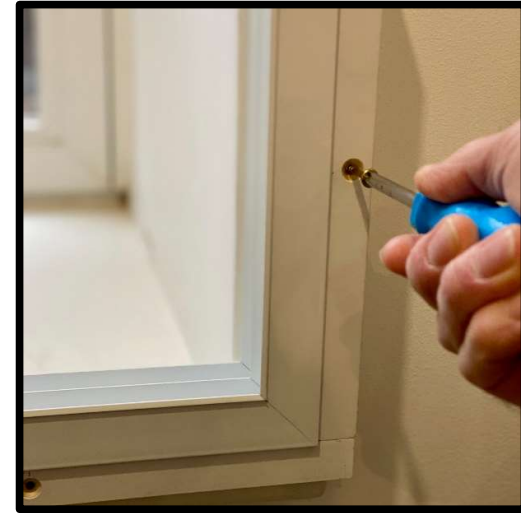
Face Fixed – Surface Mounted Around Reveal
