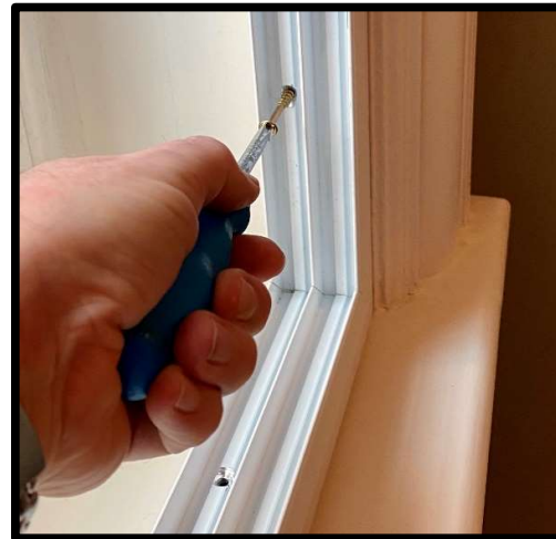
Reveal Fix - Track Drilled
