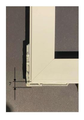
Measuring & Installation is the same as per standard instructions, namely a 10mm tolerance deduction to aperture sizes for frame build size. Packing as required for levelling & positioning. Over-trimming the gap to finish and seal.
